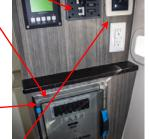
16 To dim the controller digital displays at night press the "Mode" button and the up arrow buttons on the controllers simultaneously.
