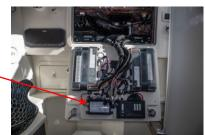
1 Ensure that the 12 volt "House" battery voltage is adequate (at least 12 volts) to power The Czone system.
