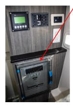
The ACOI is in the stateroom on the aft wall below the manual A.C. source select circuit breaker panel.
