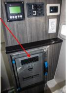
12 Ensure that the "Water Heater" circuit breaker is on in the Czone system.
