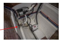
1 Ensure that the sewage tank discharge seacock is open.
