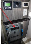
12 Ensure that the "Water Heater" circuit breaker is on in the Czone system.
