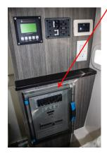
The ACOI is in the stateroom on the aft wall below the manual A.C. source select circuit breaker panel.
