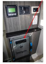
11The Czone Volts display indicates the voltage coming through to the circuit groups on the A.C. panel. The voltage should read between 110 and 120 Volts to safely operate the 120 volt equipment.
