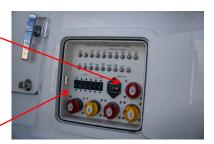
4 Ensure that the "Elect" (to feed the fuse block for the monitors and other electronics) 50a, "COI 1" (to feed COI1 D.C. Loads) 100 a, "COI 2" (to feed COI2 D.C. loads) 100 a, "OI" (LROI 20a), and "C6" (5a Output Interface) manual circuit breakers are on at the main D.C. panel. These circuit breakers feed the D.C. loads and NMEA 2000 bus of the Czone system.
