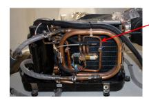
service the main deck. These are fed raw water by two dedicated 115 volt Dometic 336183 115 VAC raw water pumps. The condensate is collected in the pan under the units
