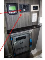
the way by turning off the circuit breaker labeled "Generator" as necessary to turn on the circuit breaker labeled "Shore".
