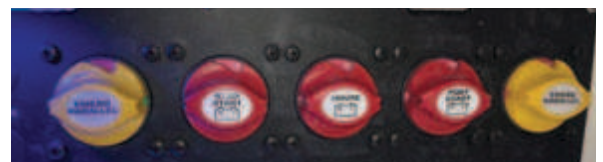
The photo above shows the battery management panel.
